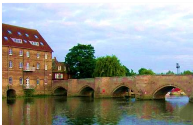
Huntingdon – Old Bridge
